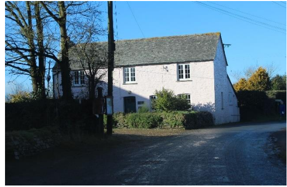
Figure 2: an example of a traditional building in the parish, showing typical proportions, detailing and characteristics. This property has rendered elevations which, as is stone and slate hanging, is a common feature in the area. Note how this property relates to the highway.
