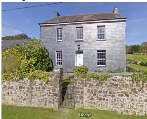
Figure 6: A larger detached dwelling in Langore showing traditional proportions and slate-hanging
