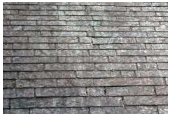
Figure 9 Silver grey natural slate in diminishing courses is typical of roofs in the Parish and contribute greatly to its character
